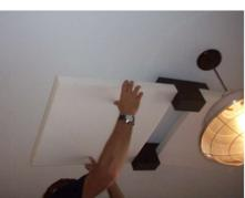
such as metal roof decks, use a positive fastening system. Attach standoffs to flutes of deck with self-tapping screws and large washers. Adhere panels to standoffs; putty knife application is recommended.
