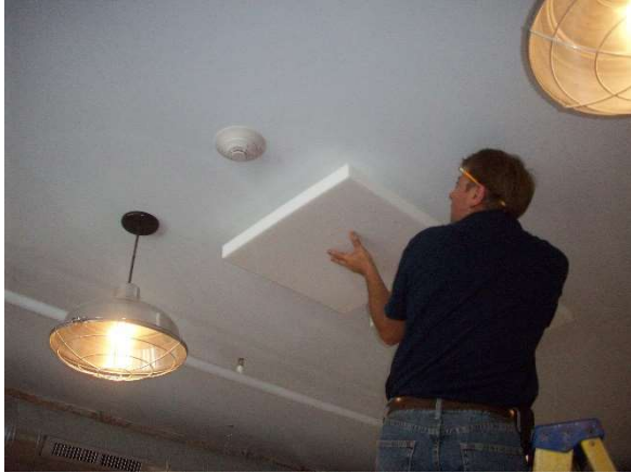
Figure 1: Gypsum board ceiling during installation
