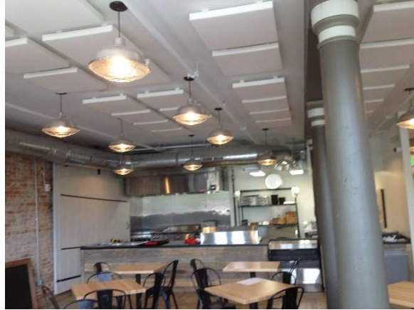
Figure 2: Dining and prep area after installation
